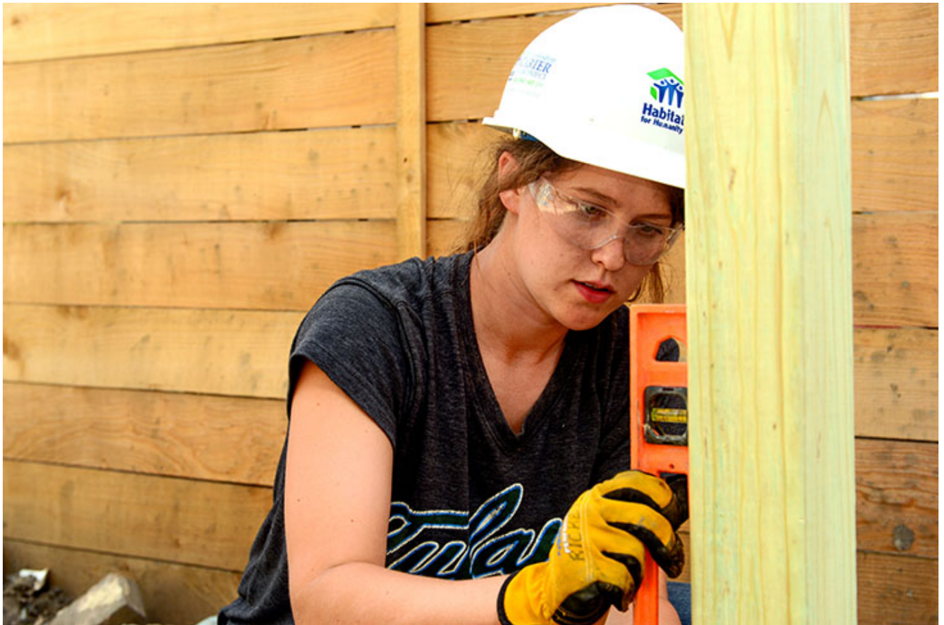
Ashley Ricketson builds the platform for the air-conditioning unit.
