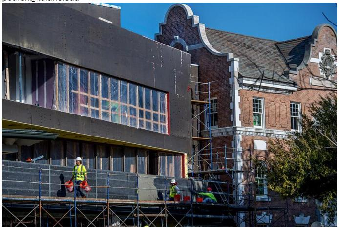
Workers begin plastering the exterior of the addition to Mussafer Hall on the uptown campus. The original building, built in 1902 as Richardson Dormitory, has undergone significant plaster and masonry work to highlight the structure's architectural details.
