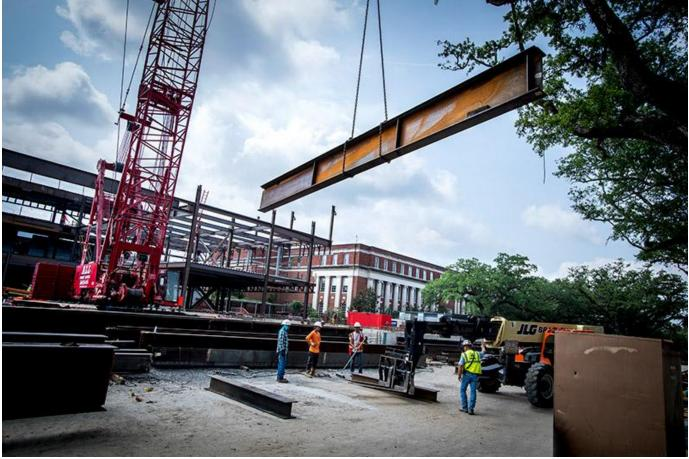
A steel beam moves slowly overhead during construction of <u>The Commons</u> on the uptown campus. Located where the Berger Family Lawn meets Newcomb Place, the new three-story structure will include a 58,000-square-foot dining facility as well as a 19,000-square-foot space for the <u>Newcomb College Institute</u>. Joseph Merrick Jones Hall is in the background.
