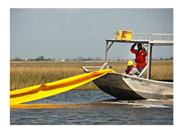
Contractors haul in oil containment boom in Bay Bourbeux, La., to reposition it. Crews work 12-hour days maintaining, repositioning and deploying boom to prevent the spread of oil into marsh grass in Terrebonne Parish. (Coast Guard photo by Petty Officer 2nd Class John D. Miller)
