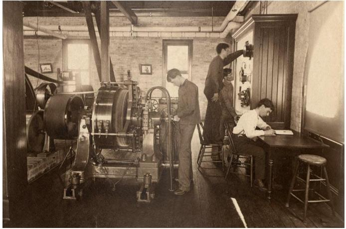
Senior electrical engineering students work with a Siemens & Halske four pole machine in the dynamo laboratory located in the engineering building, which was part of the Tulane University College of Technology around the turn of the century.
