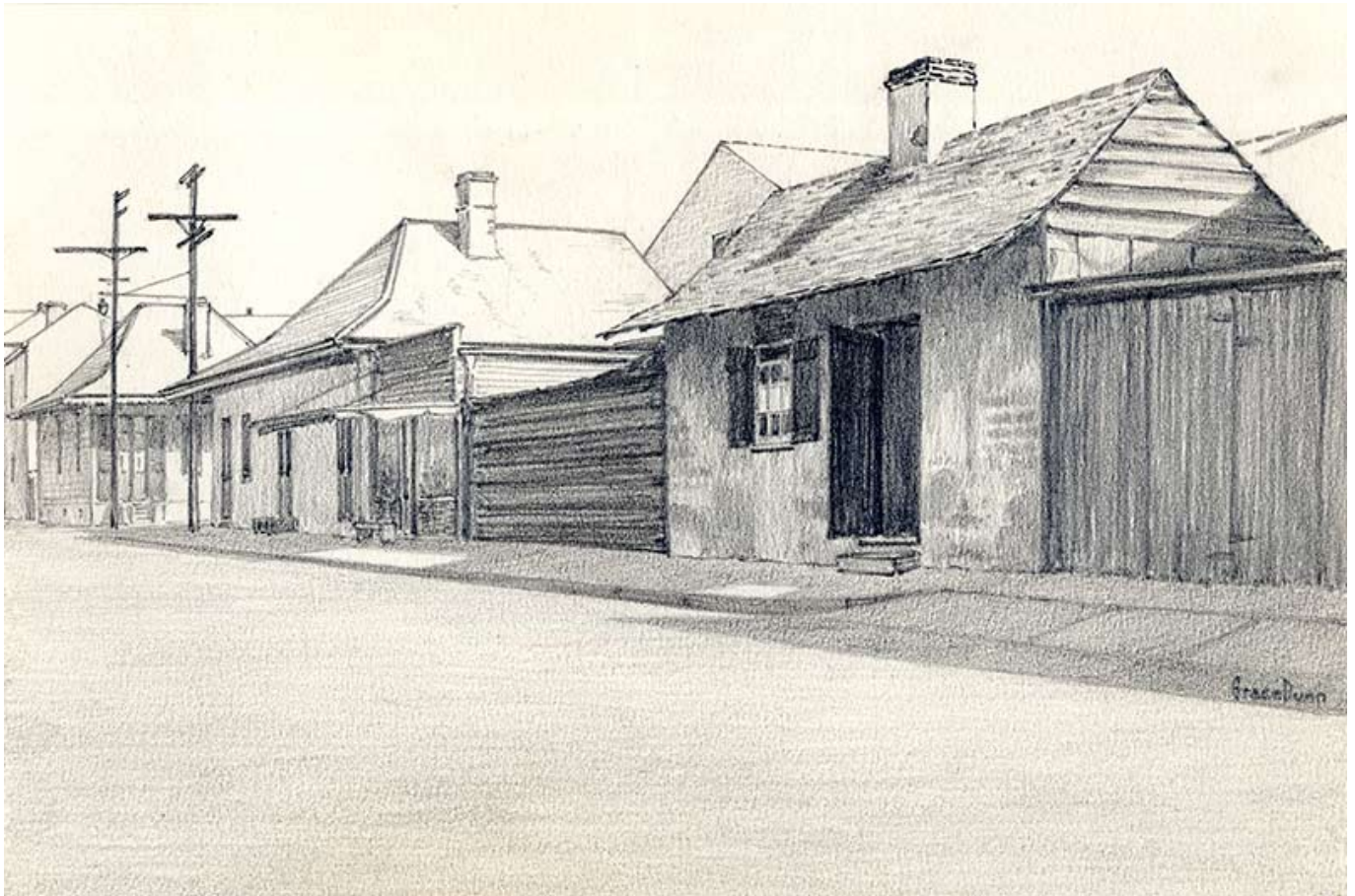
This pencil drawing by Grace Dunn shows the 700 block of South Liberty Street in New Orleans ca. 1930s. (Photo from Southeastern Architectural Archive, Special Collections Division, Tulane University Libraries)
