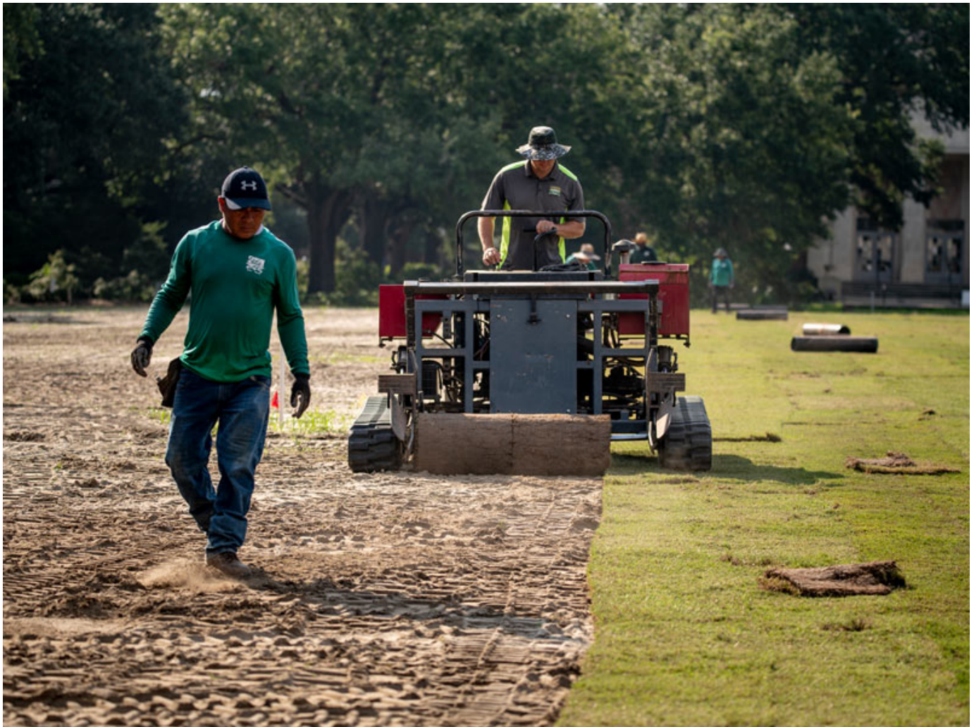
New sod is placed on Berger Family Lawn. The quads on the uptown campus were refurbished after the deconstruction of 13 temporary buildings that included classrooms and a Dining Pavilion. The additional structures were erected to provide more spaces for social distancing within classroom environments. (Photo by Paula Burch-Celentano)
