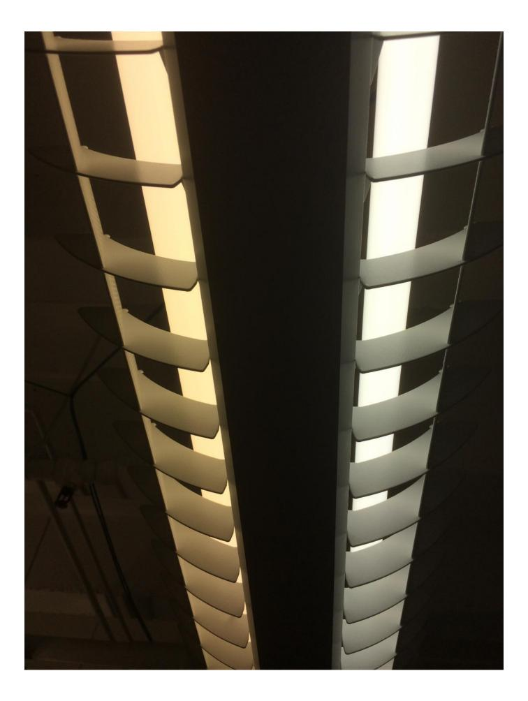
The light emitted from a Phillips state-of-the-art, solid state tunable blue-enriched LED light bulb during daytime may have more beneficial effects on health compared with a Phillips standard cool white fluorescent bulb. The standard fluorescent bulb is pictured at left and the blue-enriched bulb is at right. (Photo provided by the Laboratory of Chrono-Neuroendocrine Oncology)
