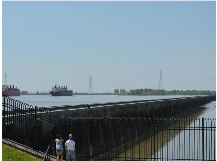
The Bonnet Carré Spillway allows flood waters from the Mississippi River to flow into Lake Pontchartrain and then into the Gulf of Mexico. It has been opened 16 times since its construction in 1937 — four times since March 2018. (Photo by Jacques Hebert)
