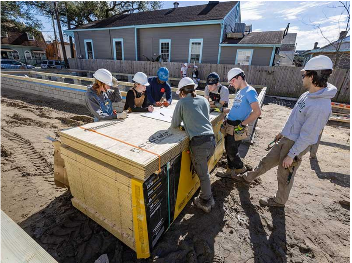
Architecture students Quinn Kelsey, left, Le'Bryant Bell, center, and Ethan Lewis, right, check a floor plank during construction of a home. (Photo by Rusty Costanza) Students go over plans for a home under construction with Sara Allen Harper, front left. (Photo by Rusty Costanza)
