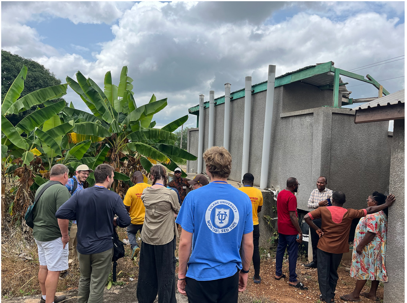
Tulane EWB joined members of HCDP Ghana and Sokode-Ando community representatives to assess composting toilet facilities in nearby Ho, Ghana. (Photo provided by Tulane Engineers Without Borders)
