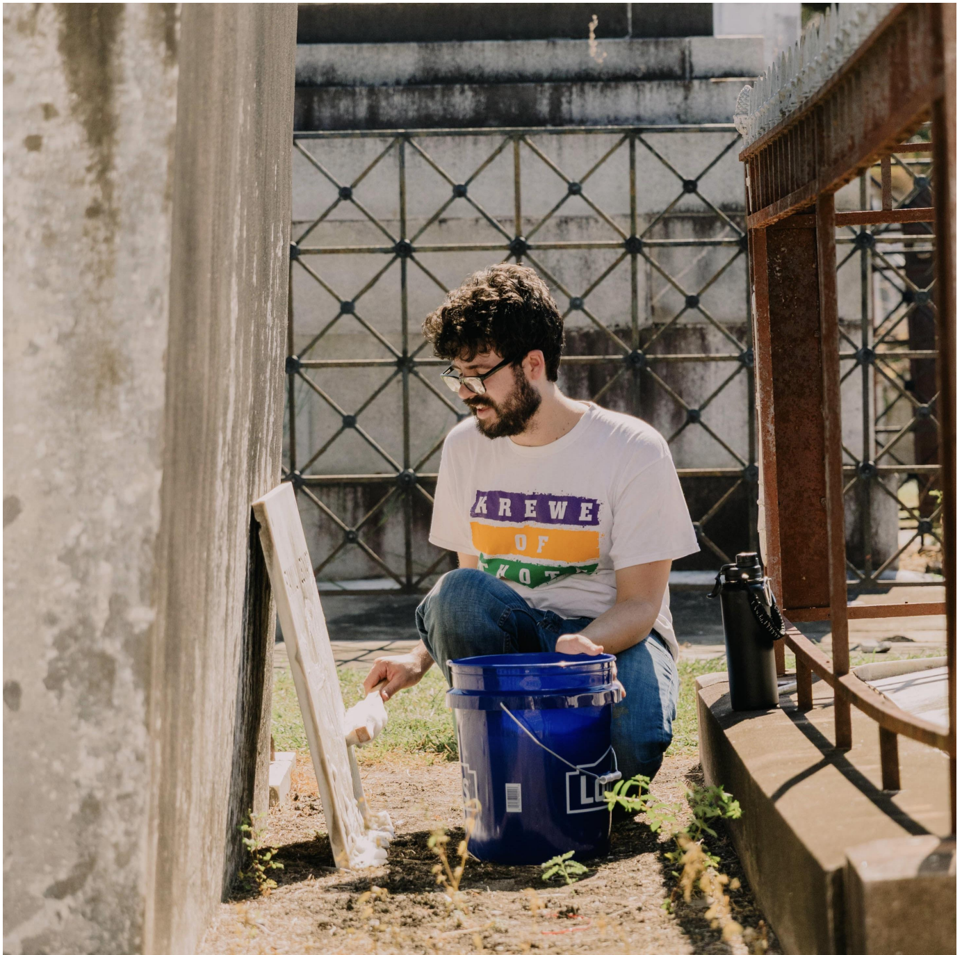
Preservation student Stone DuVernay was among a group of students from the School of Architecture and Built Environment who helped to restore graves under the instruction of program director Heather Veneziano. (Photo by Catherine Restrepo)
