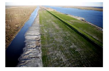
Seepage caused by underground flow of water is the likely cause of the network of channels scouring the levees along the Mississippi River-Gulf Outlet Canal, a Tulane scientist says. (Photos from Kyle M. Straub)
