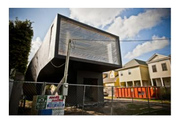
Large windows at front and back are designed to provide a panoramic view. The exterior, now with black waterproofing, will have wood cladding.
