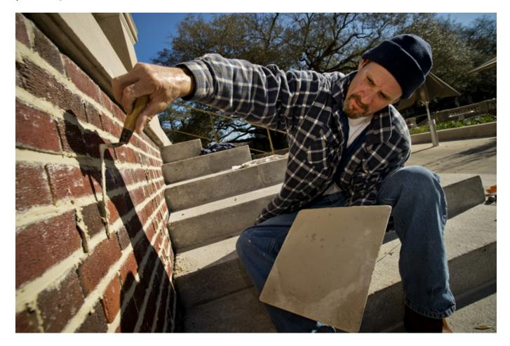
David Imbraguglio applies new mortar to the front entrance of Newcomb Hall. The mortar is visually consistent to that used in the newly constructed Benenson Plaza.
