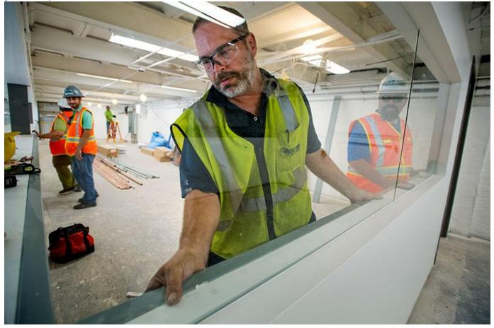
Steve Tramonte, an electrician with H.Rocker Electric, installs wiremold in the soonto-be-completed <u>Maker Space</u> on Tulane's uptown campus. Located in the old machine shop on Engineering Road, the facility offers direct vehicle access, adequate power, high ceilings, compressed air, and features multiple modern prototyping tools such as laser cutters, water jet cutters, and 3-D printers.
